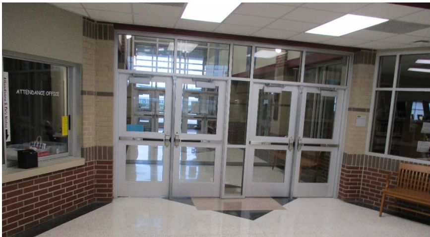
Photograph 1. Example of a Secured Vestibule
