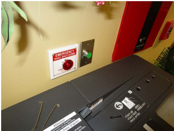
Photograph 5. Emergency HVAC Shut-Down
